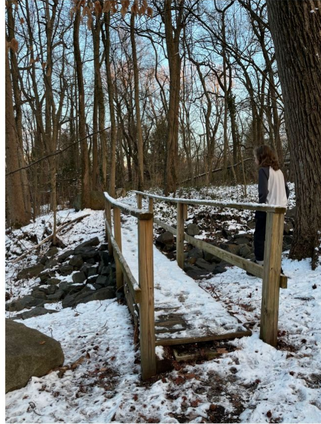
Existing conditions / view of bridge
